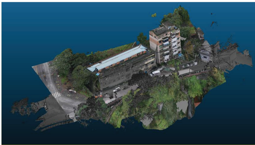
Figure 14. The integrated 3D point cloud that combines the UAV point cloud and the MMS point cloud.
